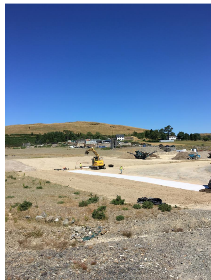
Figure 4. The full extent of the geosynthetic clay liner once deployed.
