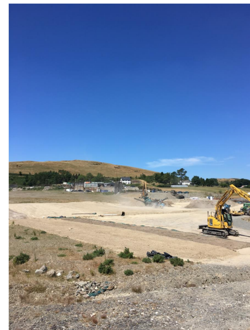
Figure 4. The full extent of the geosynthetic clay liner once deployed.
